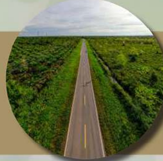
Jalan Road Infrastructure
